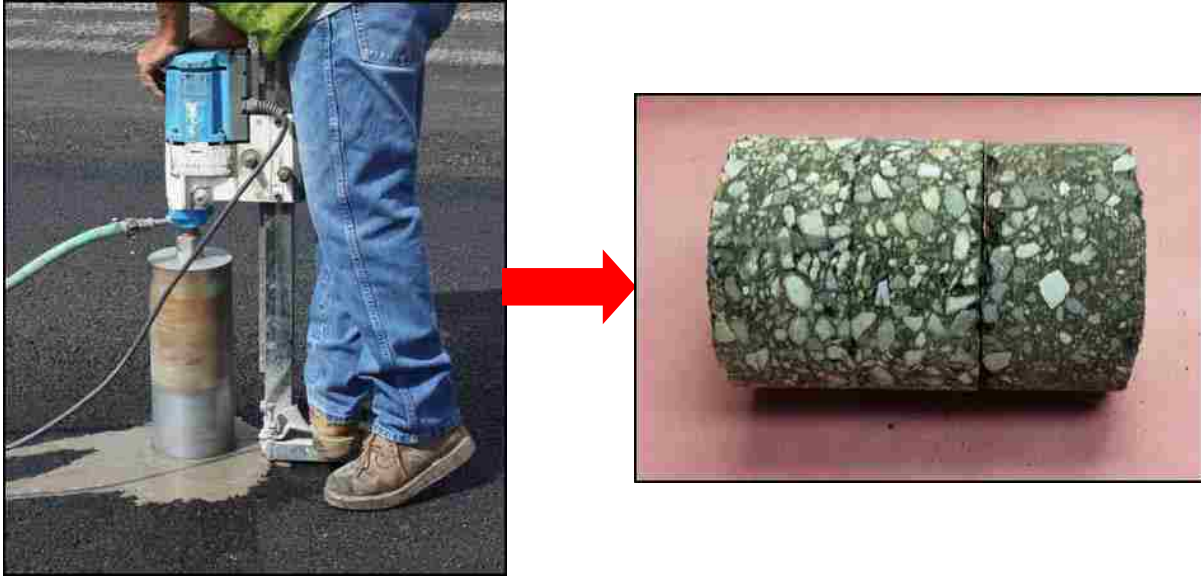
Figure 3.13 Extraction of field-compacted AC core
